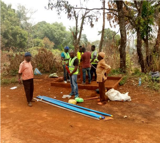
The technician arrive site with materials
