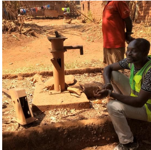
Head of the pump damaged and removed
