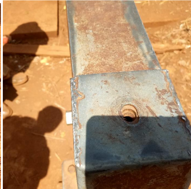
Loosed pump with no screws(boles)
