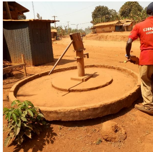
Loosed Pump: from enquiries we were told all the pipes, cylinder and rising main we
