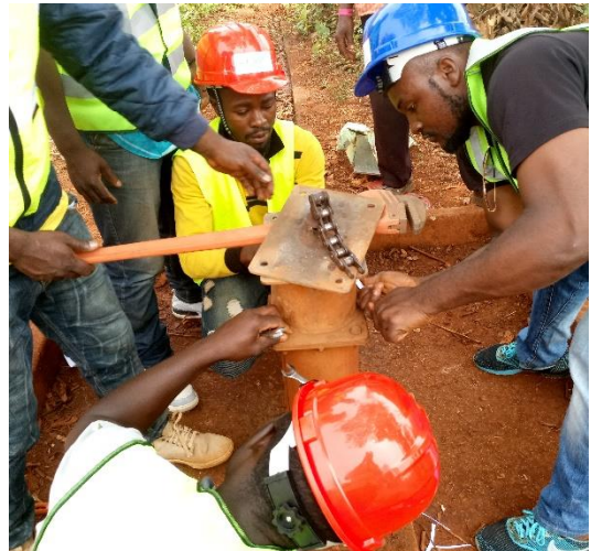
Dismounting and repair of the head of the pump
