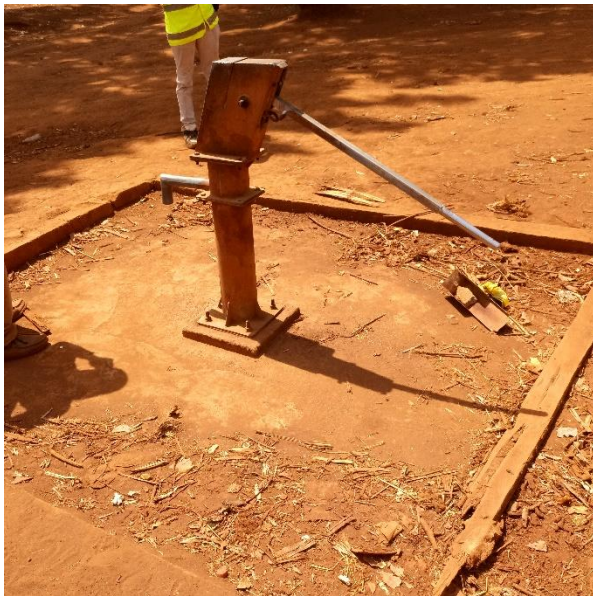
Loosed pump with no screws(boles)
