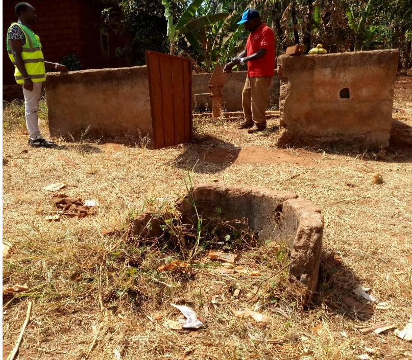
Waste pipe blocked
